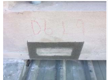
Type 2 repair done
