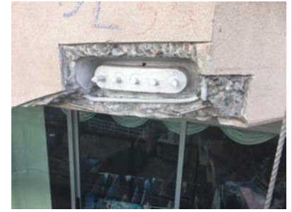
Steel preparation completed
