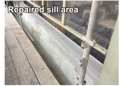
Typical window sill repair
