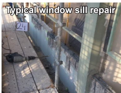
Repaired sill area
