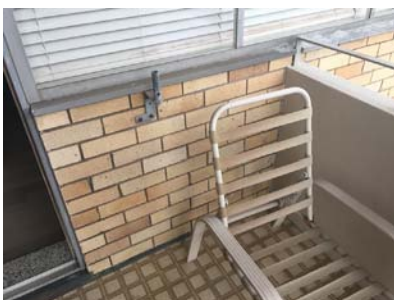
Typical balcony before
