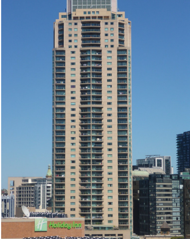
North facade before commencement
