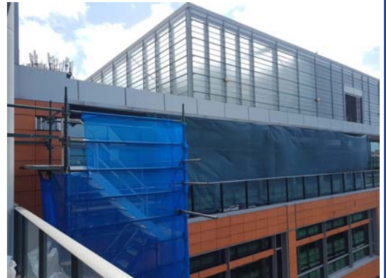
Perimeter beam formed and poured with soffit repair under way below the beam
