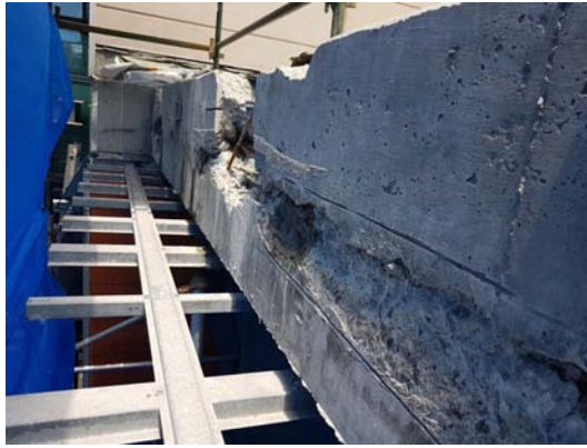
Perimeter repair area externally (left ) and internally (right)
