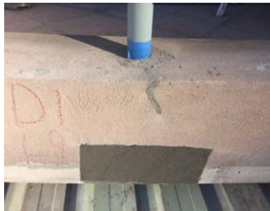
Type 1 repair done
