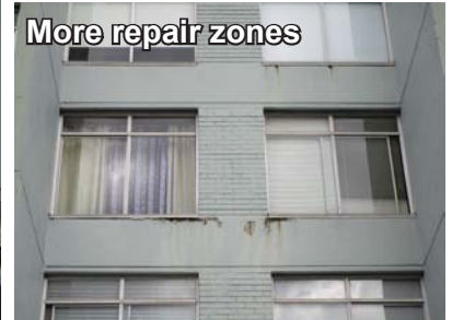
Repaired sill area
