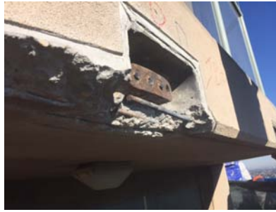
Typical stressing plate repair area
