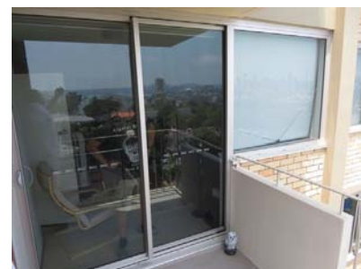
Balcony after completion
