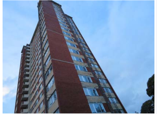
North and west under way
