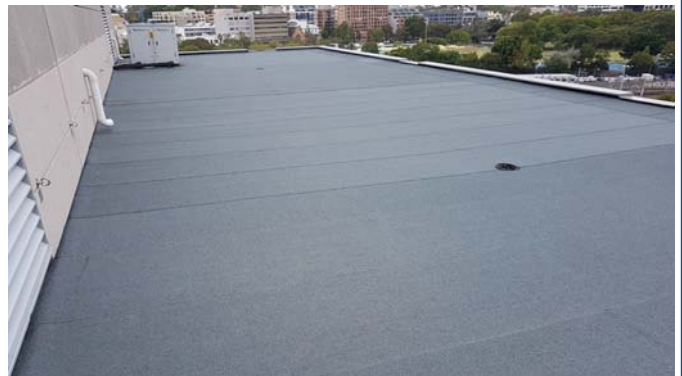
Roof area No. 26 before (left) and membrane installed and detailed (right)
