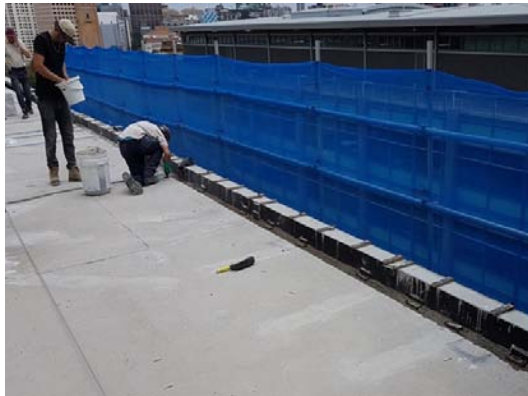
Perimeter beam formed and poured with soffit repair under way below the beam
