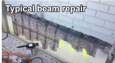
Typical sill beam repair area
