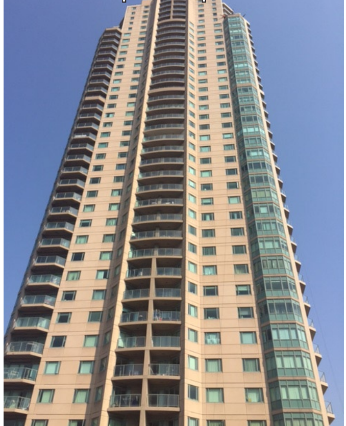
North facade repaired and protected
